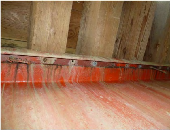
Figure 1-13: Typical deck tie to girder connection.
