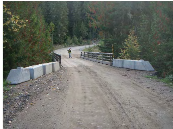
Figure 1-4: Looking towards woods end.
