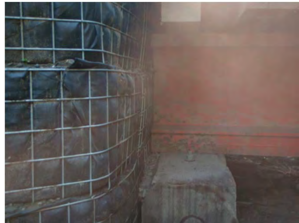
Figure 1-20: Typical ballast wall (woods end shown).
