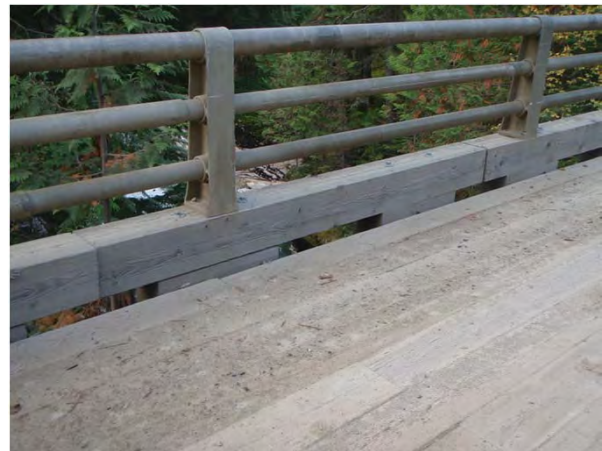
Figure 1-12: Typical curb rail and railing configuration.
