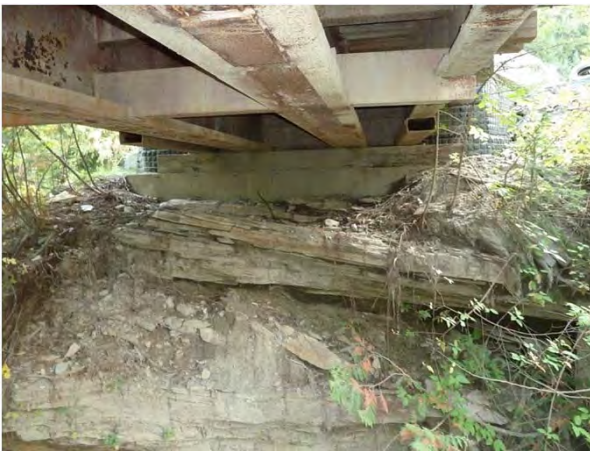
Figure 1-17: Woods end abutment.
