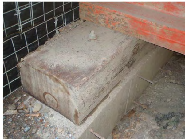
Figure 1-18: Typical sill (woods end upstream shown).
