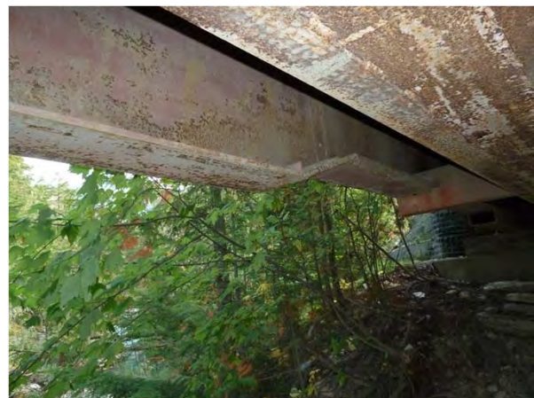
Figure 1-24: Typical end of exterior girders (woods end upstream shown).
