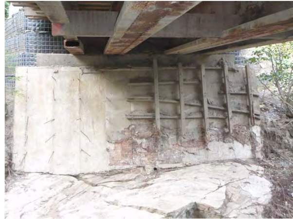
Figure 1-14: Camp end abutment.
